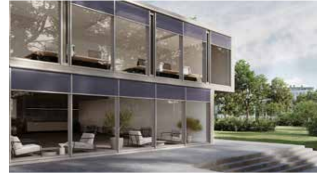
installation on the curtain wall
