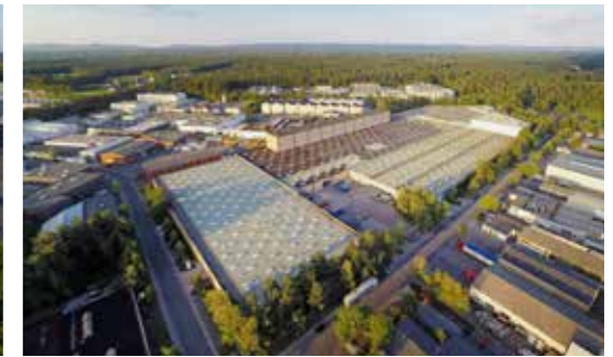
Plant II, Hövelhof, Germany
